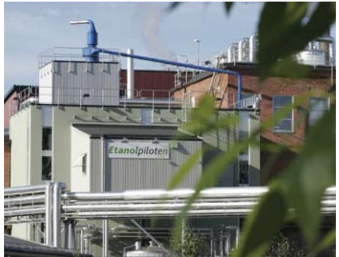
Promising for the future are biofuels produced from ligno-cellulosic feedstocks. Pilotplant for bioethanol from wood in Örnsköldsvik. (Photo: SEKAB)
